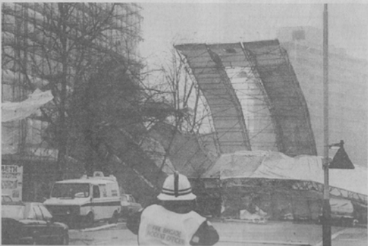
Ripped apart: Scaffolding from a block of flats in Briston crashing down yesterday as the fiercest winds since October 1987 brought London to a standstill.
